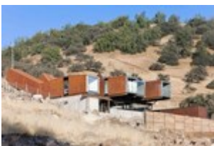
"Caterpillar House", Santiago de Chile, Chile, by Sebastian Irarrazaval architects, 2013.
